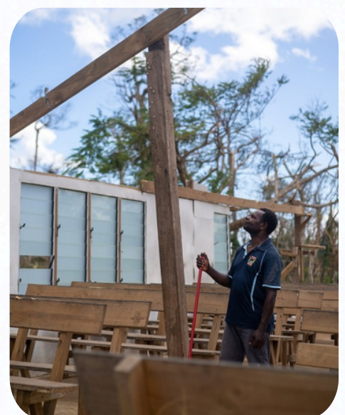
Church leader examining damaged church. Source: VANGO.
