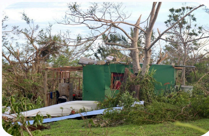
Home destroyed by Cyclone Pam in 2015. Source: Adventist Development and Relief Agency.
