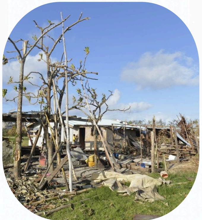
Damaged home after Cyclone Pam in 2015. Source: New Zealand High Commission, Vanuatu.
